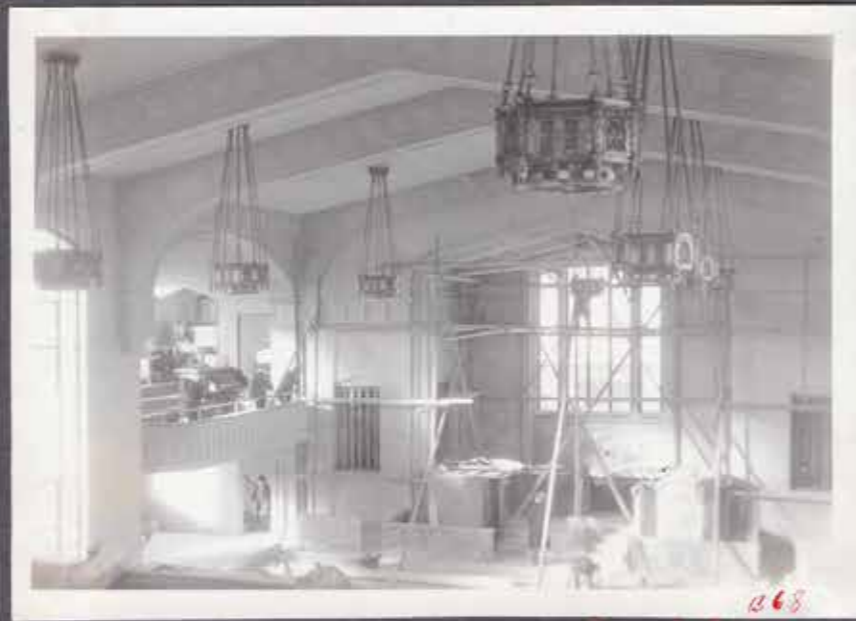
North Japan College Church under Construction
