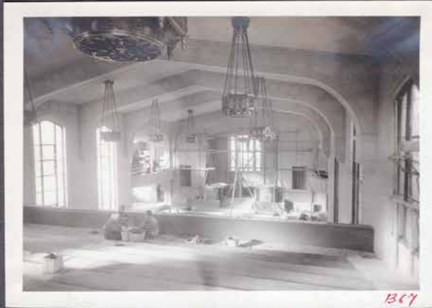
Tohoku Gakuin Chapel under Construction
